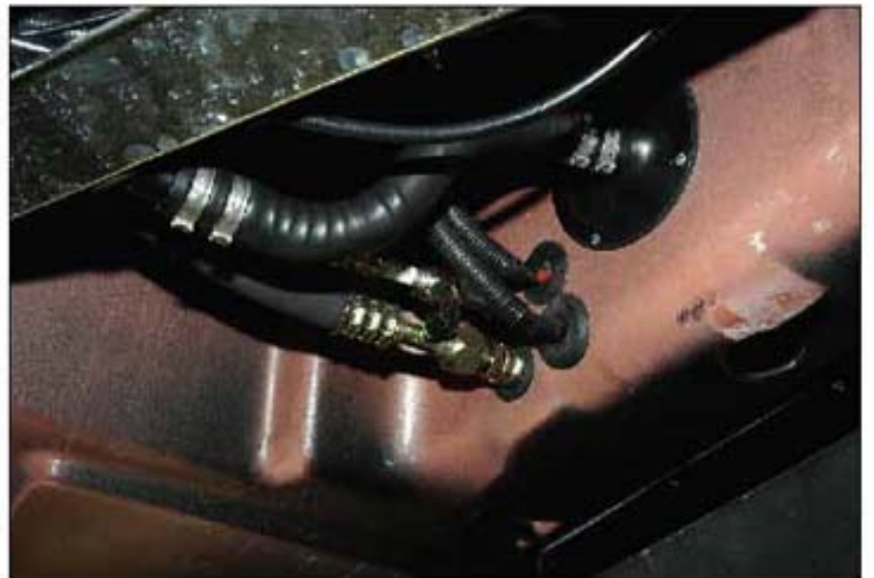
012 UNDERSIDE VIEW OF AC PIPES
