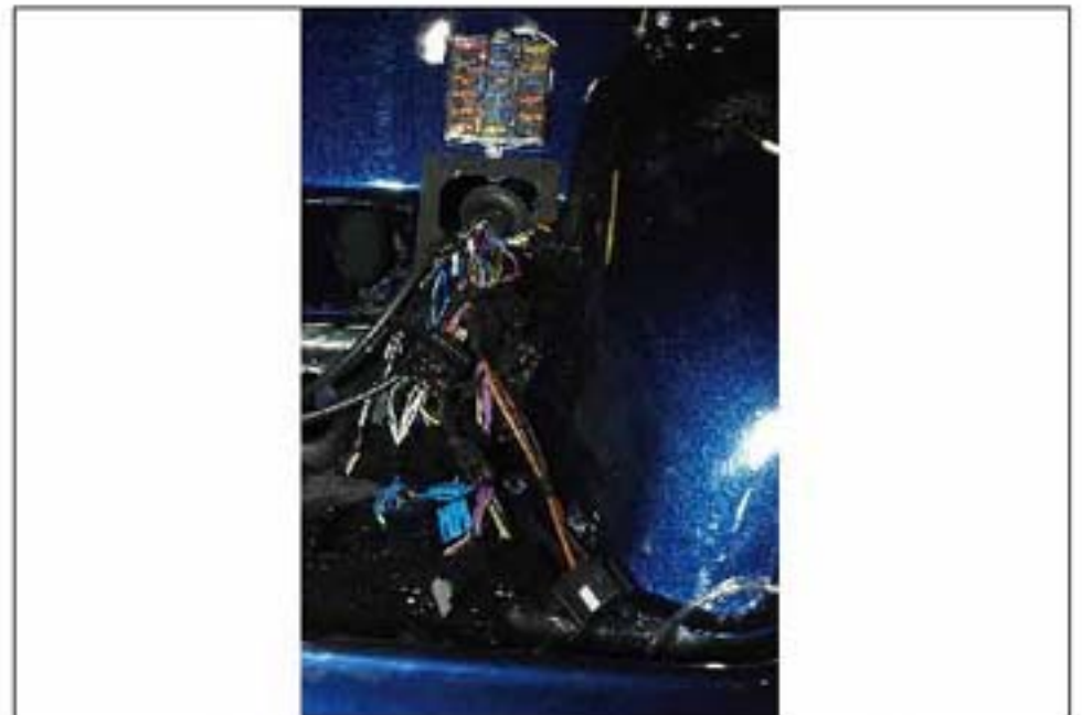
004 FRONT VIEW OF FUSE BOX & RELAY AREA
