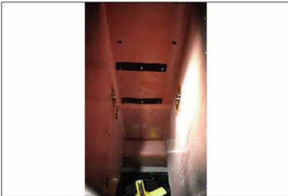
011 UNDERSIDE VIEW OF BODY CENTRE TUNNEL
