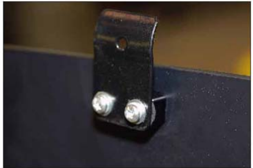
018 VIEW OF ROOF PANEL SECURING TONGUE
